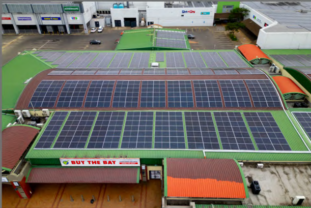
Recycling company in Pinetown, KZN: 200kW Grid Tied PV Solution, with generator intergration.
